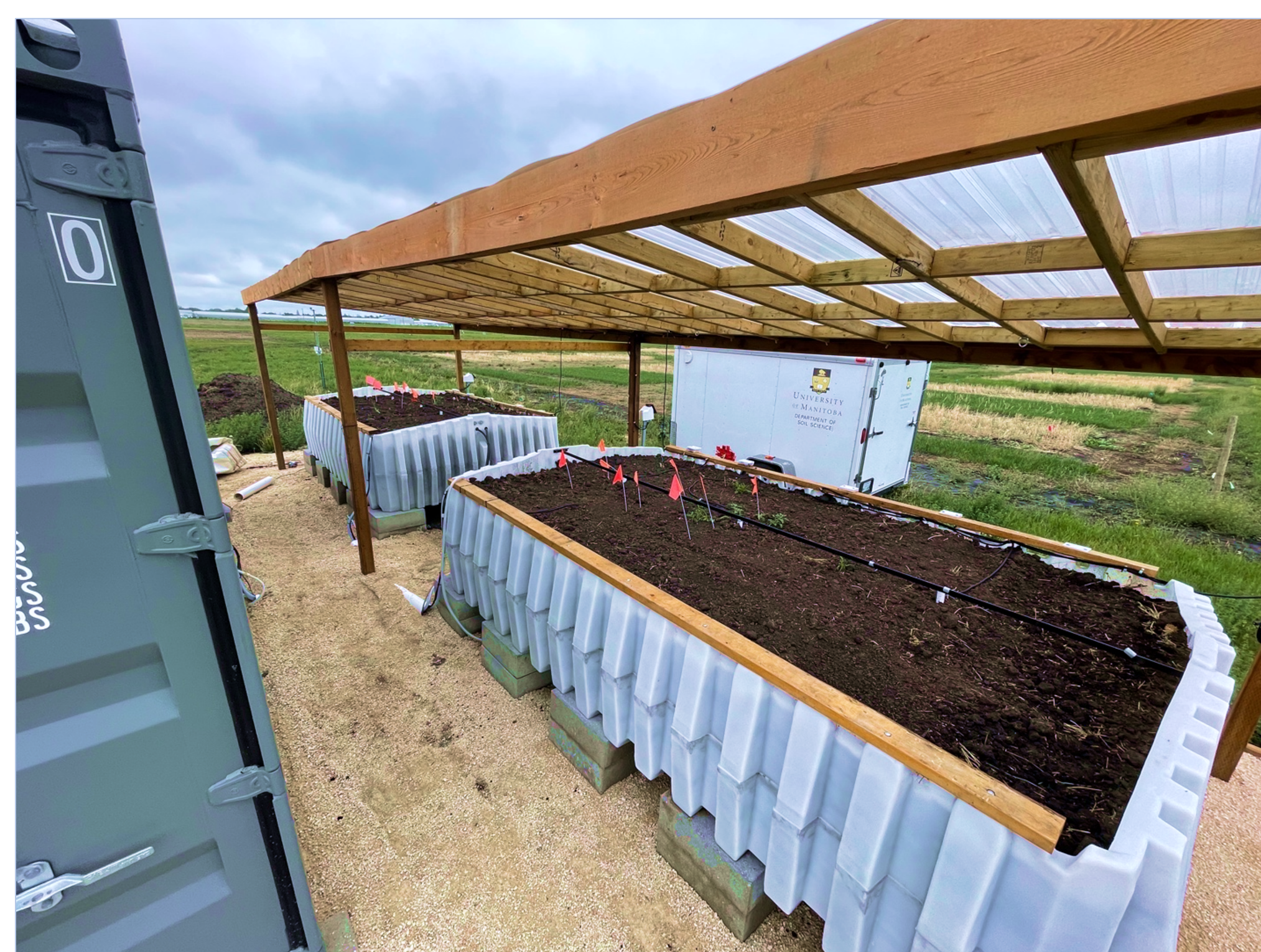
Figure 3. The two-celled biobed that became operational at the Ian Morrison Research Farm in Carman, MB in 2020
