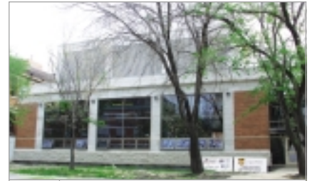
7 McQuade Structures Lab (completed 2003)
