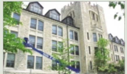
4 Tier Building (being renovated)
