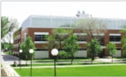
8 East Wing Addition of Agriculture Building (completed 1998)
