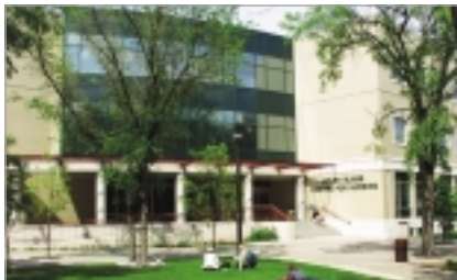
12 Helen Glass Centre for Nursing (completed 1999)
